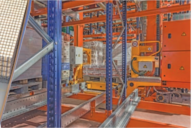
Image of an automated warehouse with Pallet Shuttle consisting of five load levels served by a stacker crane.
